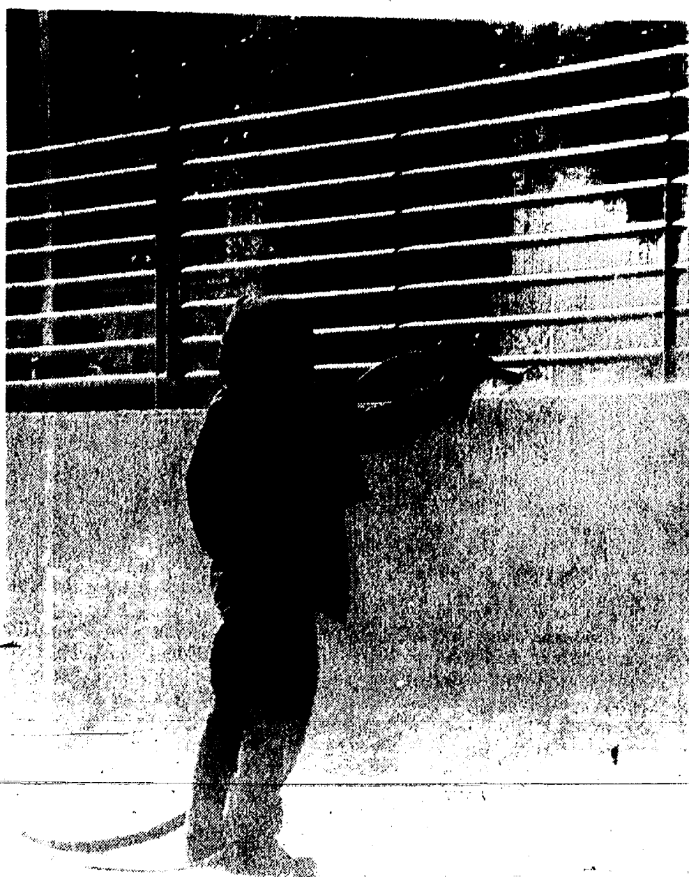
THE RETAINING WALL in the new downtown parking lot gets a sandblasting to improve its appearance. It's all part of the downtown streetscape project.
